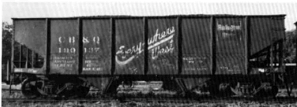
CB&Q HT-1 190137, one of the original 1926 AC&F cars, displays a post-1937 paint scheme in this 1940's view at Omaha. The horizontal seam in the side panels is readily evident.—Bernard Corbin photo, BRHS collection
