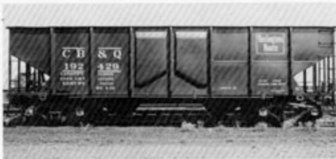
HT-2 190854 was retrofitted with aluminum side, end and slope sheets at Havelock and photographed there on Aug. 11, 1944, upon completion of the work. Note that two-piece side panels were still utilized.—CB&Q photos, Rod Masterson collection
