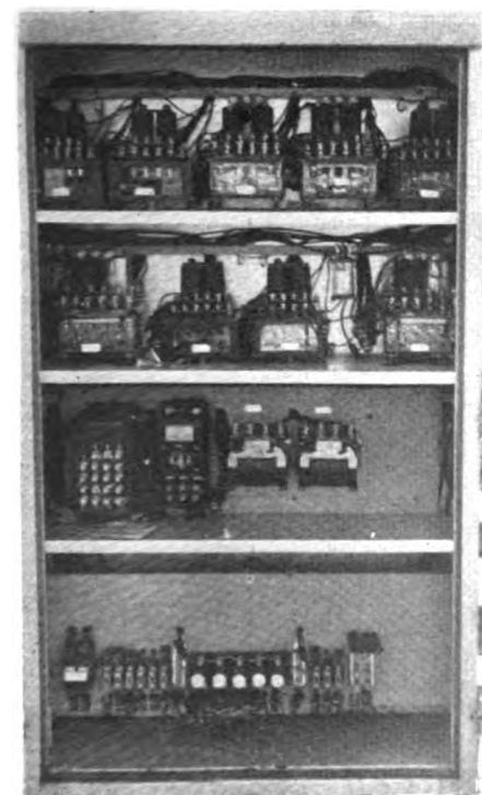
Instrument case at intermediate signal
