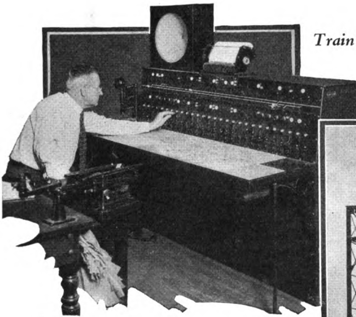
The control machine at Rochelle
