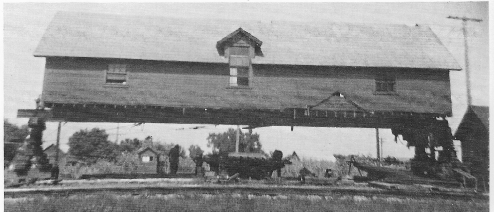
More than a dozen CB & Q two-story depots in Nebraska were reused in part by having the second-story living quarters removed intact from atop the first story. These former upper levels were then adapted as one-story structures. Such a technique was demonstrated in 1959 as, pictured above, the top story of the Mason City CB & Q depot was left suspended in air after the bottom story was torn out from under it. The second story was then lowered from its bracing onto house moving equipment for relocation. — Frank Aden photo
